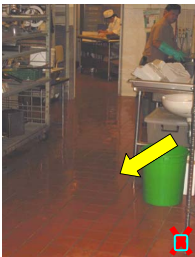
Wet floor can cause slips and falls
